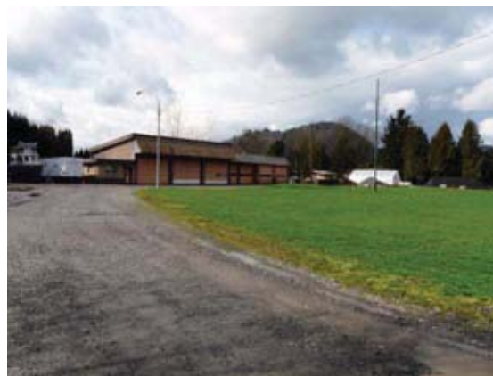
Maintenance Yard on Cheam Avenue
