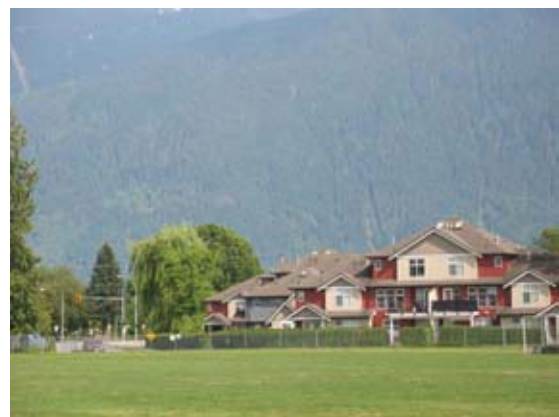
Multi-family housing adjacent to Agassiz Secondary School
